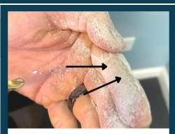
Tip: You should notice during pre-drilling, wood (darker color) will be present when backing the drill bit out, indicating you have hit a stud.
